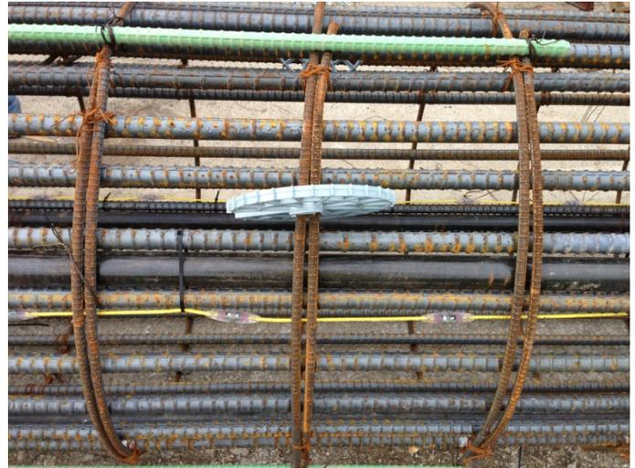
*Embedded Thermal Wire cable (yellow) attached to rebar cage*
